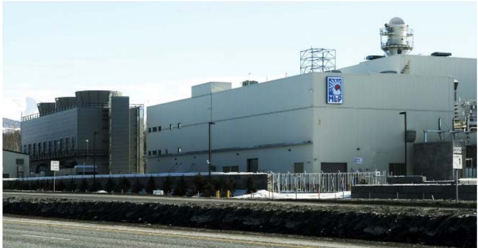
The George M. Sullivan Plant 2a along the Glenn Highway in Anchorage. (Erik Hill / ADN file photo)
